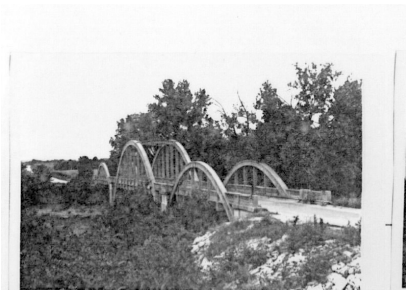
Creamery Bridge. 1979. Nimz, Dale.
